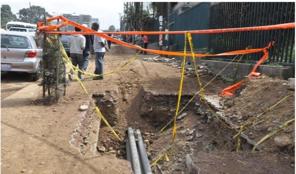
PLATE 3-2 PEDESTRIAN ROAD BLOCKED BY EXCAVATION FOR MAINTENANCE OF UTILITY LINES IN ADDIS ABABA
